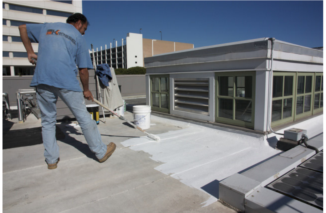
Figure 3 | Cool roof being applied to flat commercial rooftop, adjacent to photovoltaic panels
